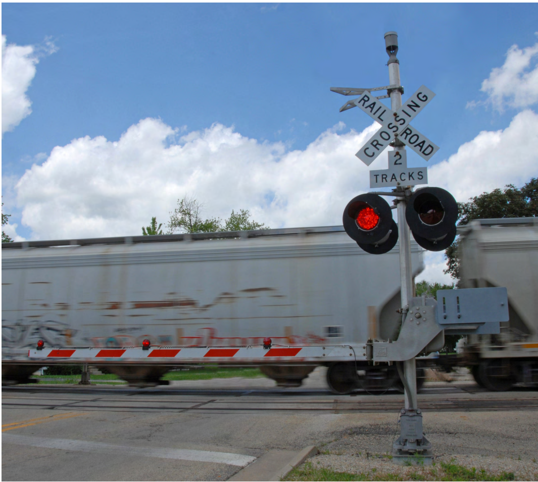
The Railway-Highway Crossings Program funds safety improvements at crossings.
