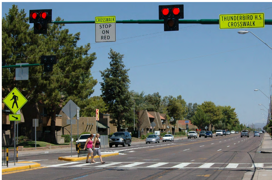
FIGURE 2-5: Pedestrian hybrid beacon (Source: pedbikeimages.org/Mike Cynecki)
